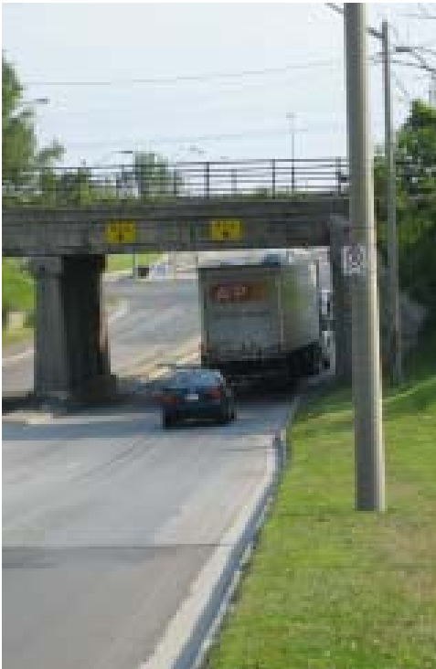
No room for pedestrians at Centennial underpass
